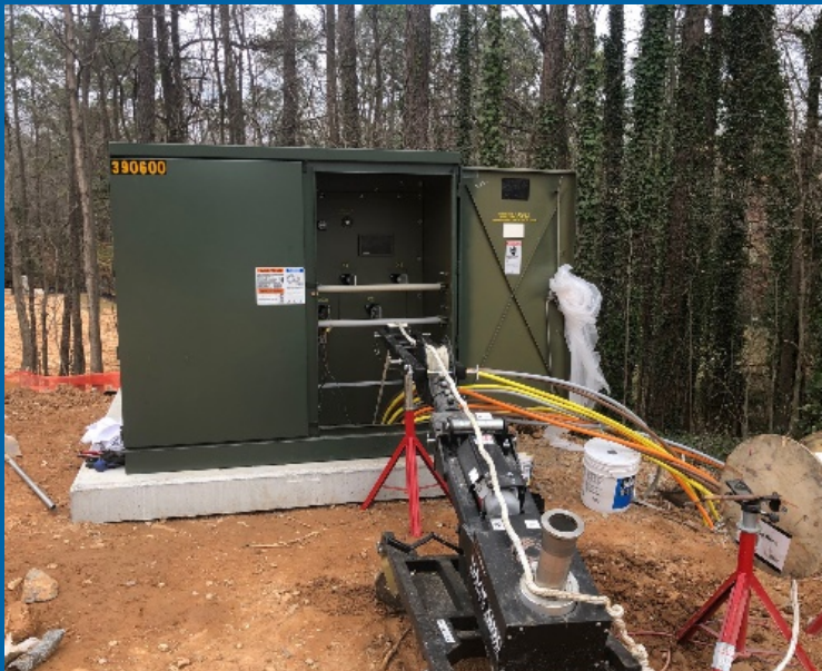
Main Feeders at New Transformer
